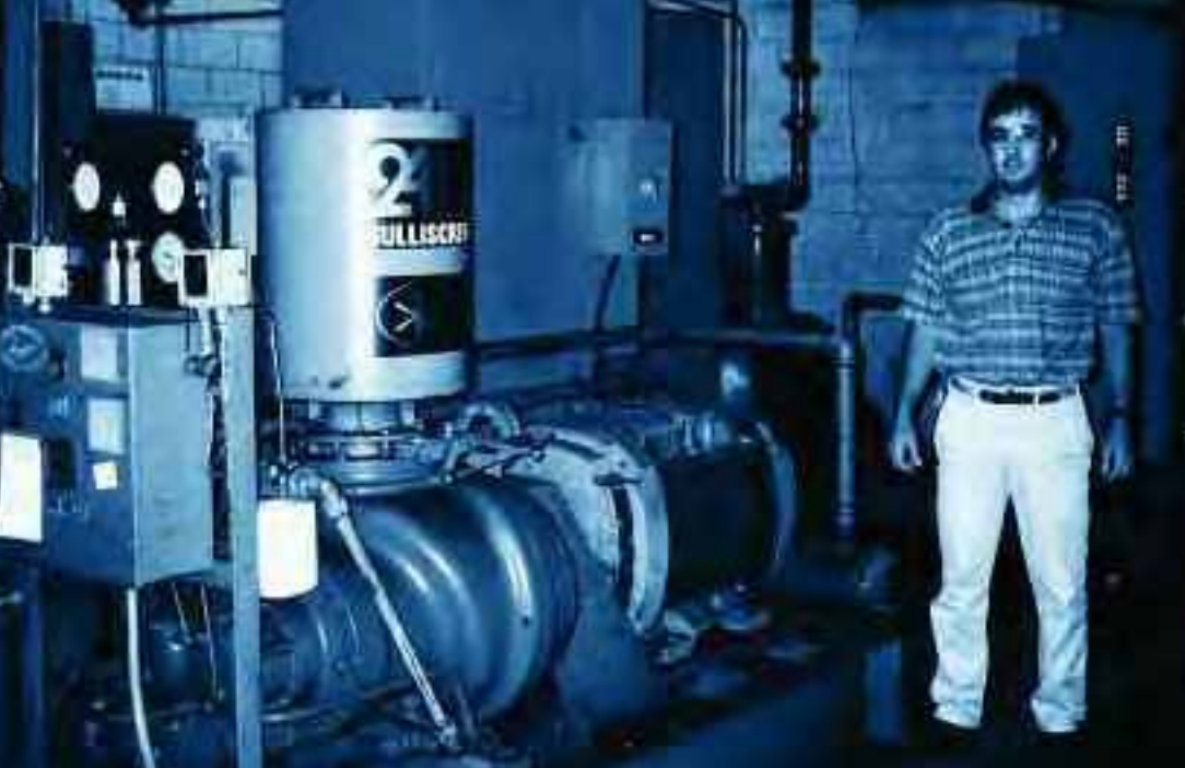
Maintenance and Facilities Engineer Alberto Koett checks a Sullair 24KT™ compressor that has been delivering oil-free air at Caribe GE for more than 25 years.
